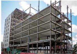
Figure 1.1(b): Frame Structure (Structuralsteel frame, n.d.)
